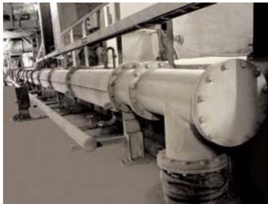
FLUIDCON transport system at Holcim plant Lägerdorf for 230 t/h cement
