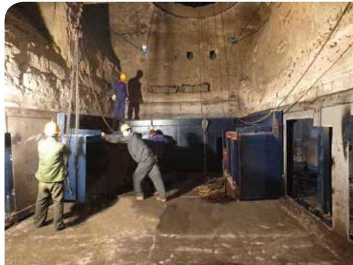
Figure 2. Positioning of the side aeration.
