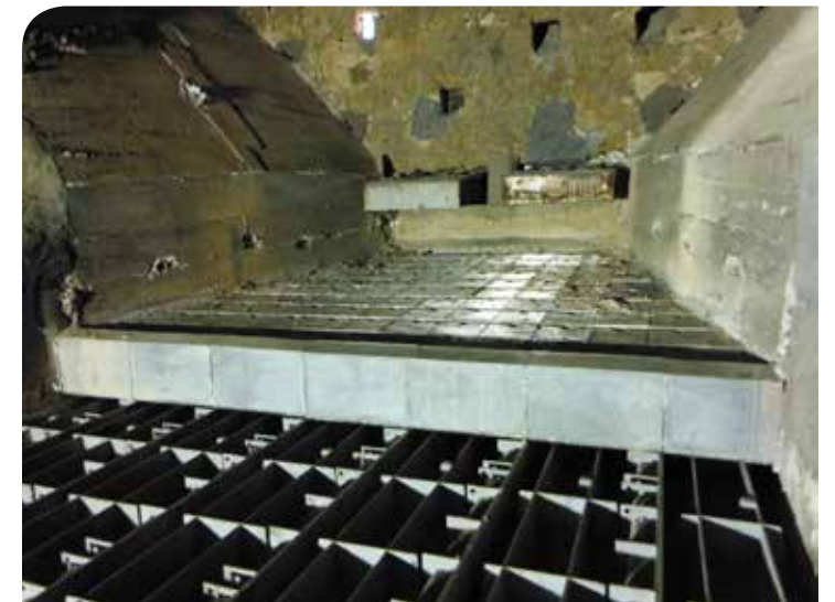
Figure 5. Transition between static inlet and lanes.
