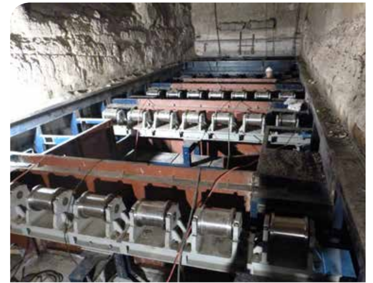
Figure 4. Cooler prepared for the installation of the lanes.
