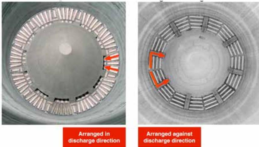
Figure 2. Radial arrangement of an EC silo (left). Tangential arrangement of an ME silo (right).
