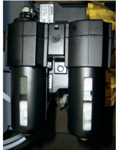
Preventive maintenance by air conditioning unit
