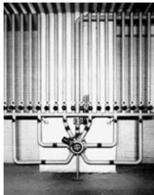
Former air distribution with mechanical distributor
