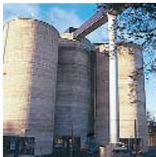
Storage Silo EC, Kantvik, Finland
