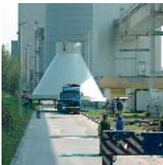
CC silo delivery on site
