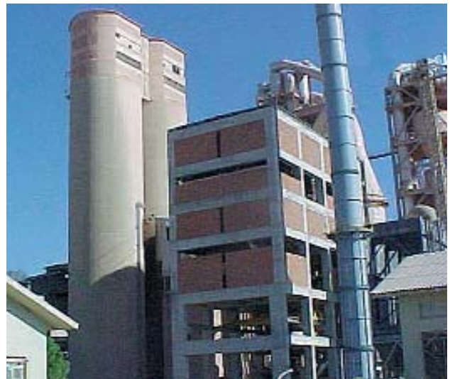
Modernization of a two-storey silo with MC silo technology, Turkey
