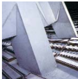
Expansion chamber - outside
