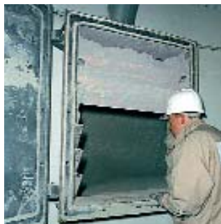
Ring channel inspection
