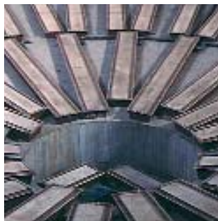
Expansion chamber - inside
