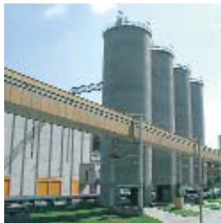
Storage Silo MF after completion, Austria
