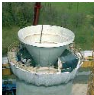
Erection of the CC silo
