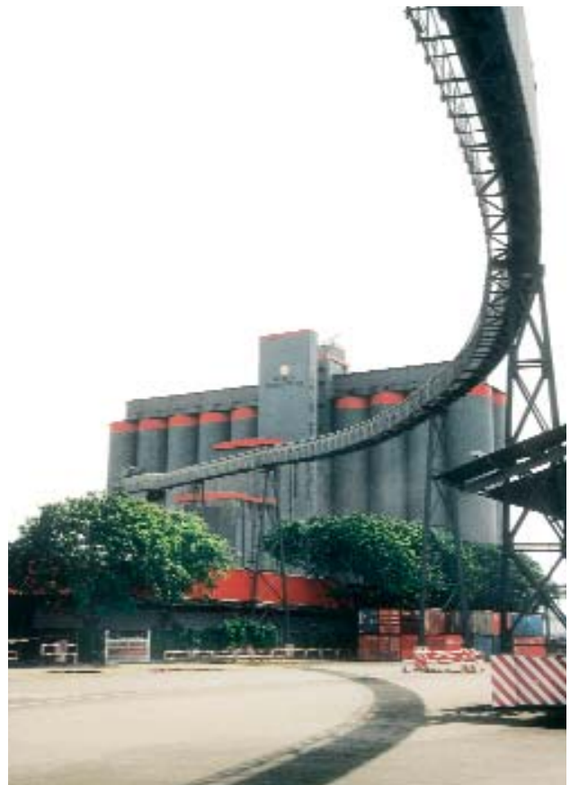
Singapore, modification of a grain terminal to a cement terminal
