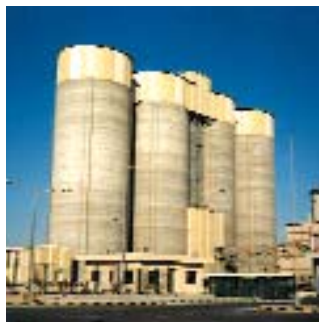
Storage Silo IC, Saudi Arabia
