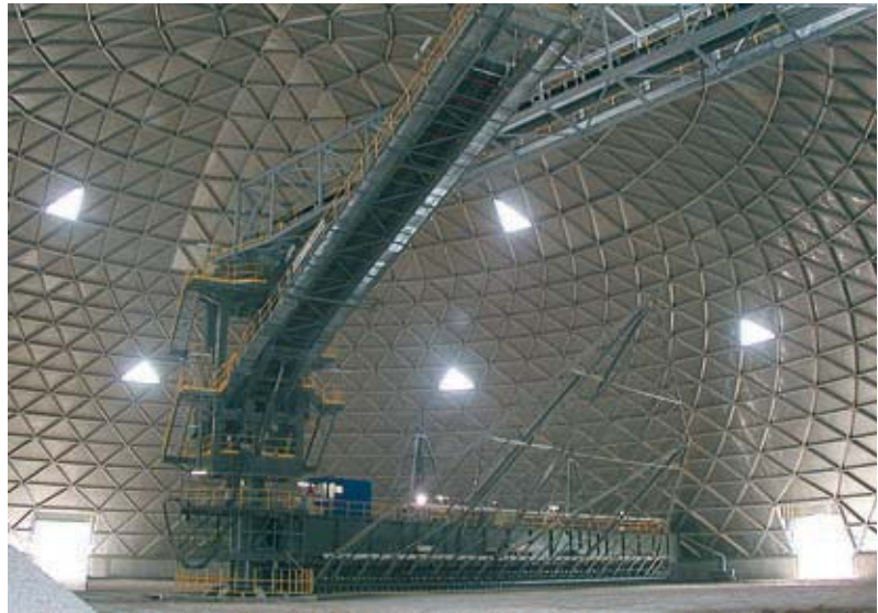
Circular blending bed for cement raw mix
