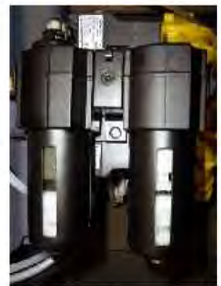
Preventive maintenance by air conditioning unit
