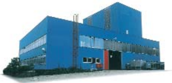
Technical Centre at Buxtehude
