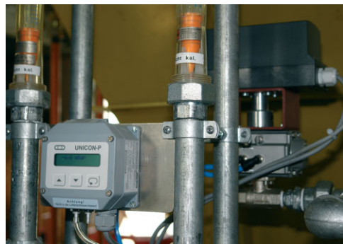
② Pressure transmitter
